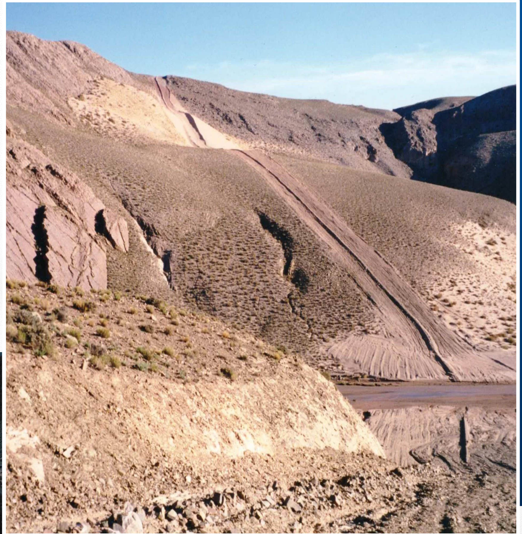
Pipeline Right-of-Way, Jujuy Province, Argentina (Elev. Approaching 4,500 m) Gas Atacama Pipeline
